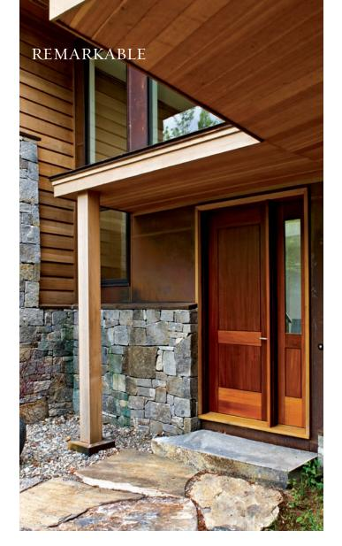
Vertical-grain Douglas fir was used for the soffit (above) and for the ceiling in the enclosed porch. The bold eaves not only help protect the house from the elements, but they also add to the natural shade provided by the neighboring trees. "The owner was drawn to the site and to the Prairie Style roof for a very practical reason," Van Dam says, "he didn't want too much sunlight."
